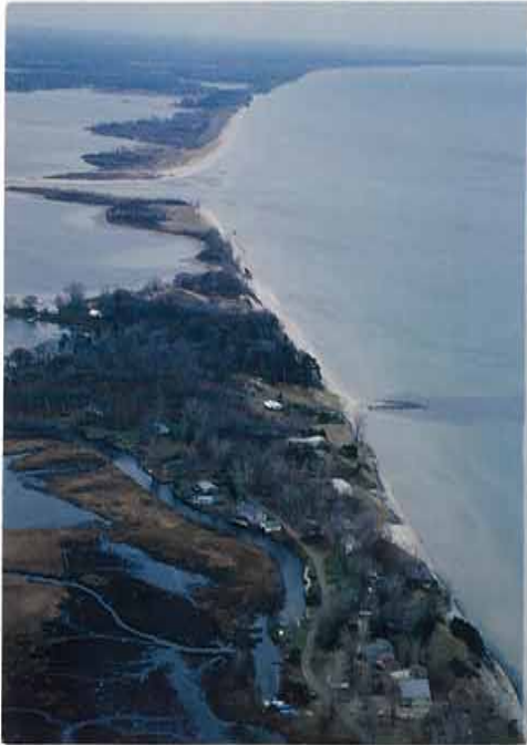
Figure 2-1: Looking south over the coastal barrier at North Pond.
