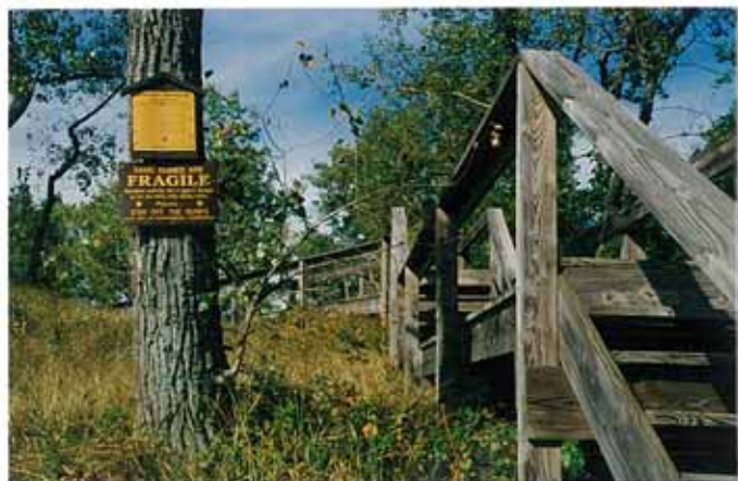
Figure 5-24: Walk-over structure in Lakeview WMA.
