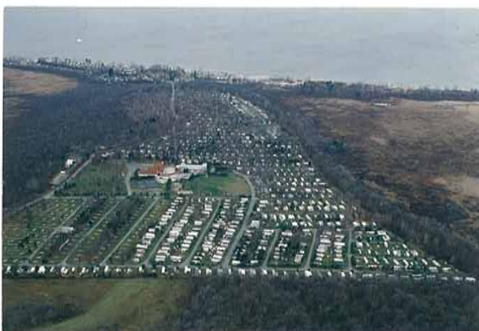
Figure 2-26: Brennan Beach campground is the most intensely developed area in the Dune and Wetland System.
