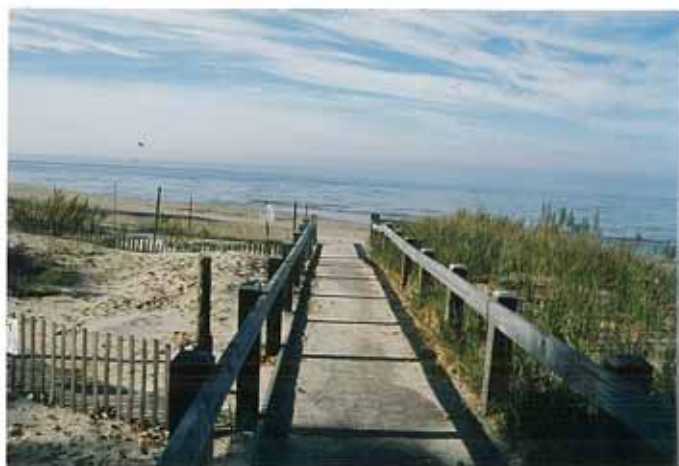
Figure 5-27: Dune walk-over at Southwick Beach State Park.
