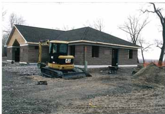
Figure 5-10: Bath-house with community room under construction at Sandy Island Beach State Park.
