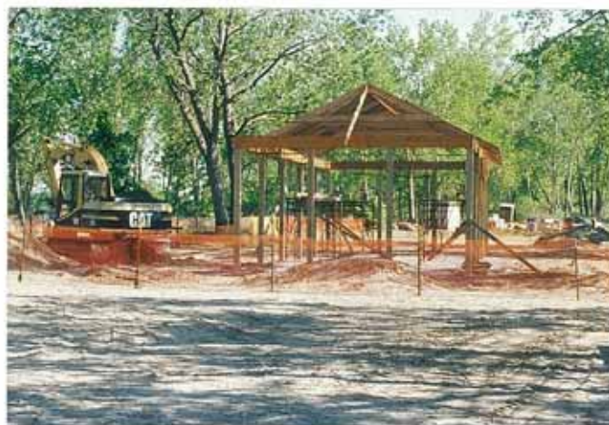
Figure 1-10: Beach pavilion under construction at Sandy Island Beach State Park.
